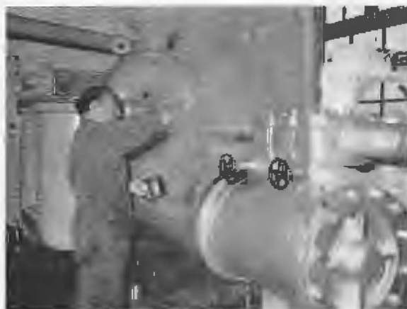
Arthur Andrew at work in the pump room of the Miramar Installation.
